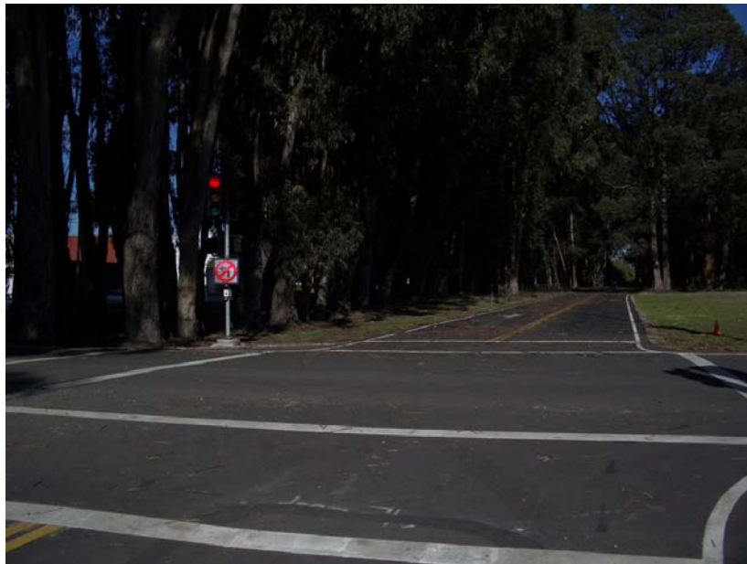
Figure 5.2 Richmond Field Station Testing Intersection
